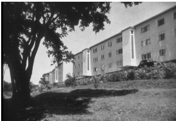
Figure 6. May's Delamere Flats Apartment Buildings, Nairobi, designed 1938-39, built 1947-51. Source: Anon. (1953), 'Flats in Nairobi, Kenya (Delamere)', Architect's Journal 117:3019 (8 January).
