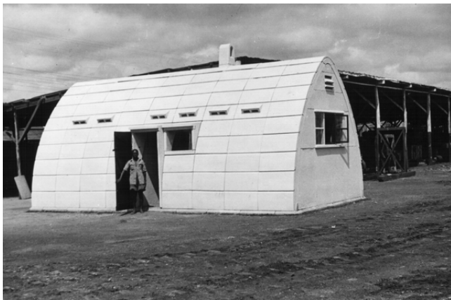
Figure 11. May's 'Hook-on-Slab' concrete-panel huts for Africans, 1945. Source: Collection of the author.
